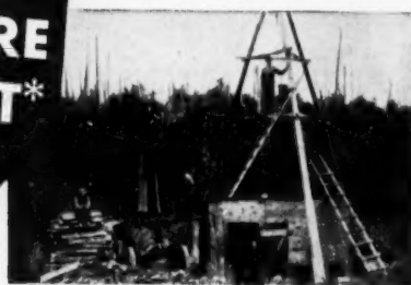
E. J. Longyear drilling first diamond drill hole on Mesabi Iron Range in 1890.
